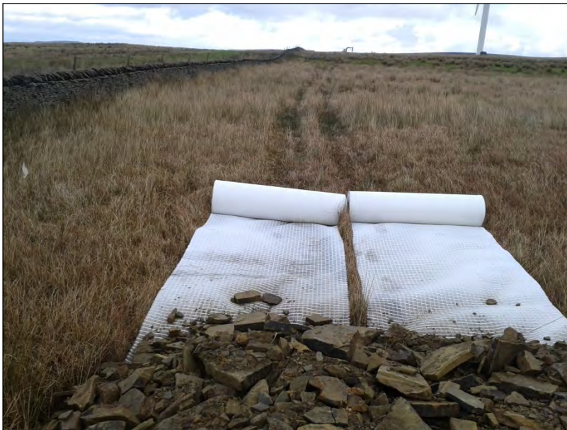
Plate 13: semi-permeable geotextile layer
